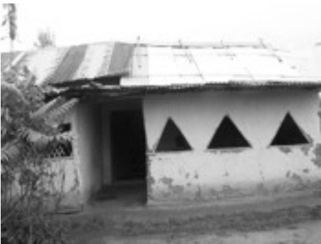
Current state of the school - six classrooms made out of mud
