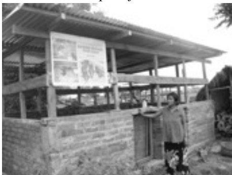
New structures built for pig farm - a community based project
